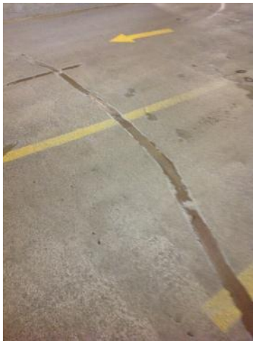
A03 – Repairs at traffic membrane in garage
