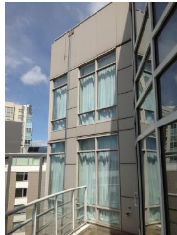
A06 – Metal panel cladding
