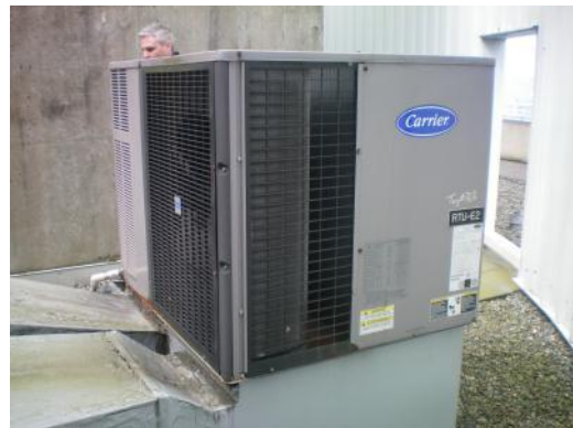
M19 – Cooling-only RTU for East Tower PH
