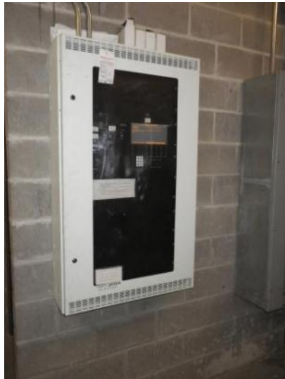
E08 – Fire alarm support panel
