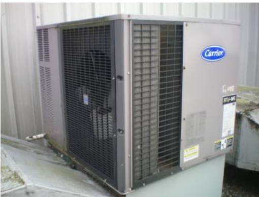
M18 – Cooling-only RTU for West Tower PH
