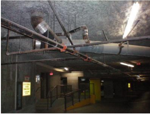
M10 – Cast iron sanitary piping in parkade
