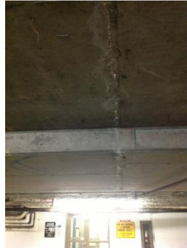
A02 – Water staining at garage ceiling
