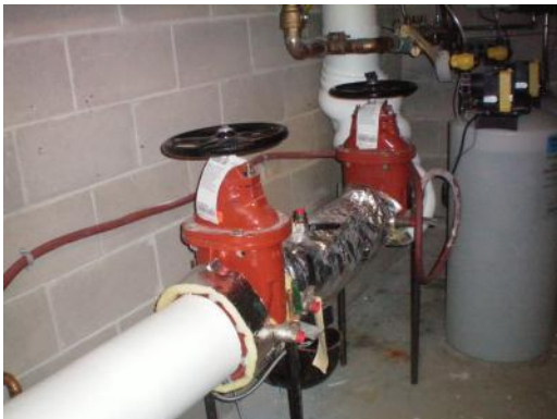
M02 – Supply branch to fire suppression systems
