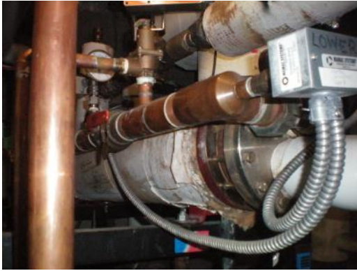
M04 – DHW heat exchanger for Lower zone
