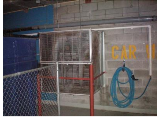
M11 – Typical exhaust fan in parkade
