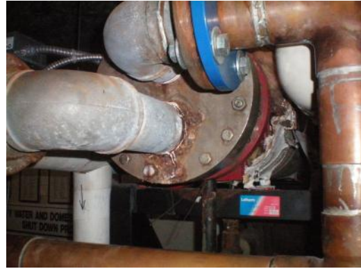
M05 – DHW heat exchanger for Upper zone
