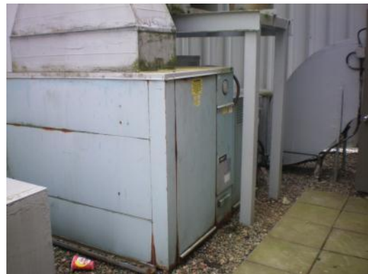
M13 – Make up air unit on the West Tower
