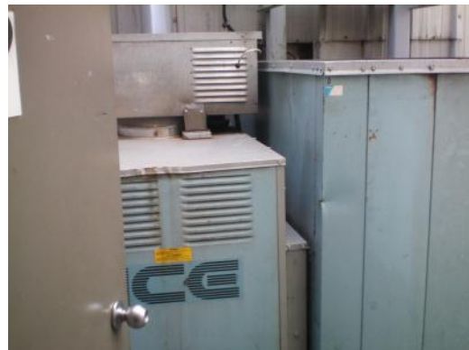
M15 – Make up air unit for East Tower upper floors
