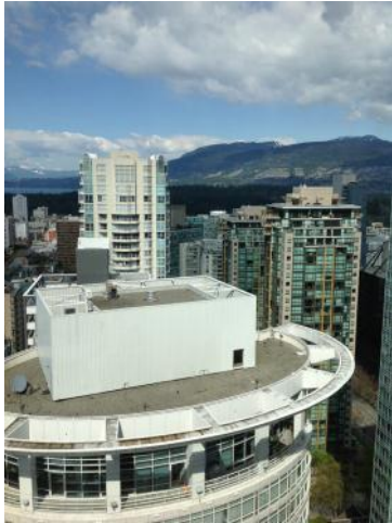
A07 – Metal clad wind screen at elevator penthouse, 1288 Alberni
