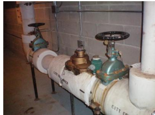
M01 – City water meter & piping
