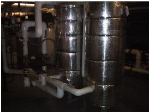
M06 – Upper level DHW storage tanks
