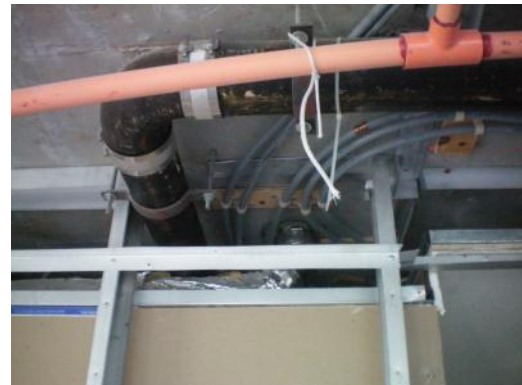
M03 – Typical polybutylene piping within suites
