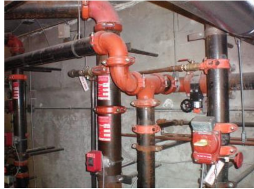
M17 – Sprinkler piping in sprinkler valve room
