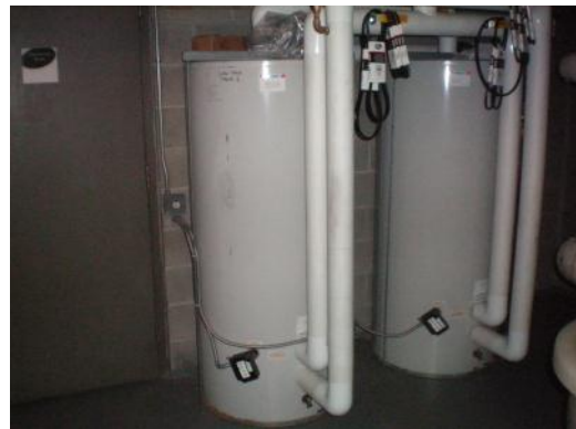
M07 – Lower level DHW storage tanks
