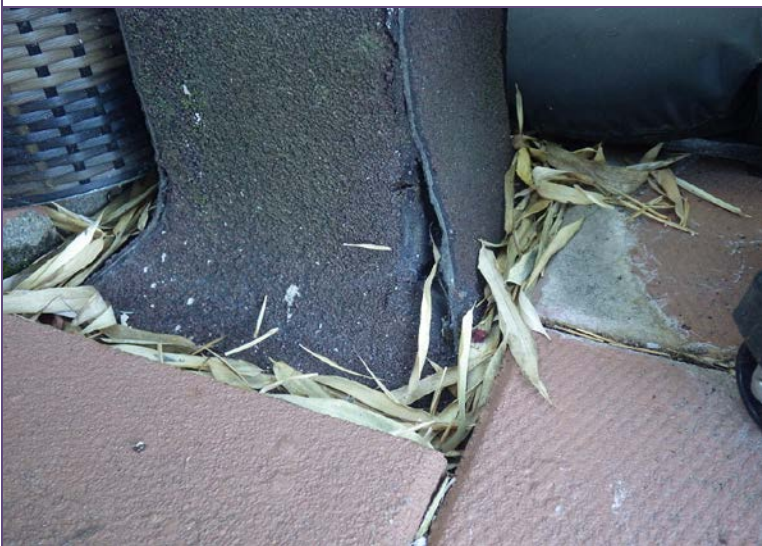
33. #803C loose stripping plies at trellis support.
